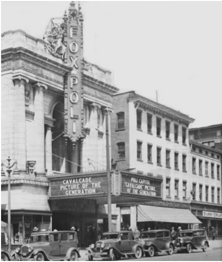
Fox Poli, Main Street, 1933. An impressive façade featured gigantic fluted columns with Ionic capitals supporting a cornice line accented by a wide frieze. A massive central arch with a recessed window achieved a three-dimensional presentation. By the early 1930s the Fox circuit had taken over the Poli chain; Fox would later be taken over by the Loew theater chain.
